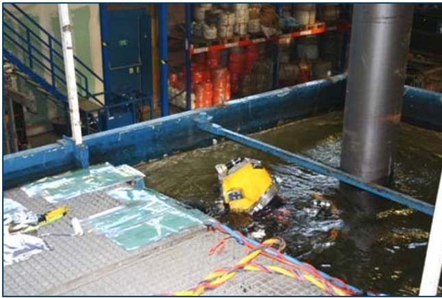
Two divers applied the STOPAQ system per sheet to the pole dummy in the diving tank during the demonstration.
